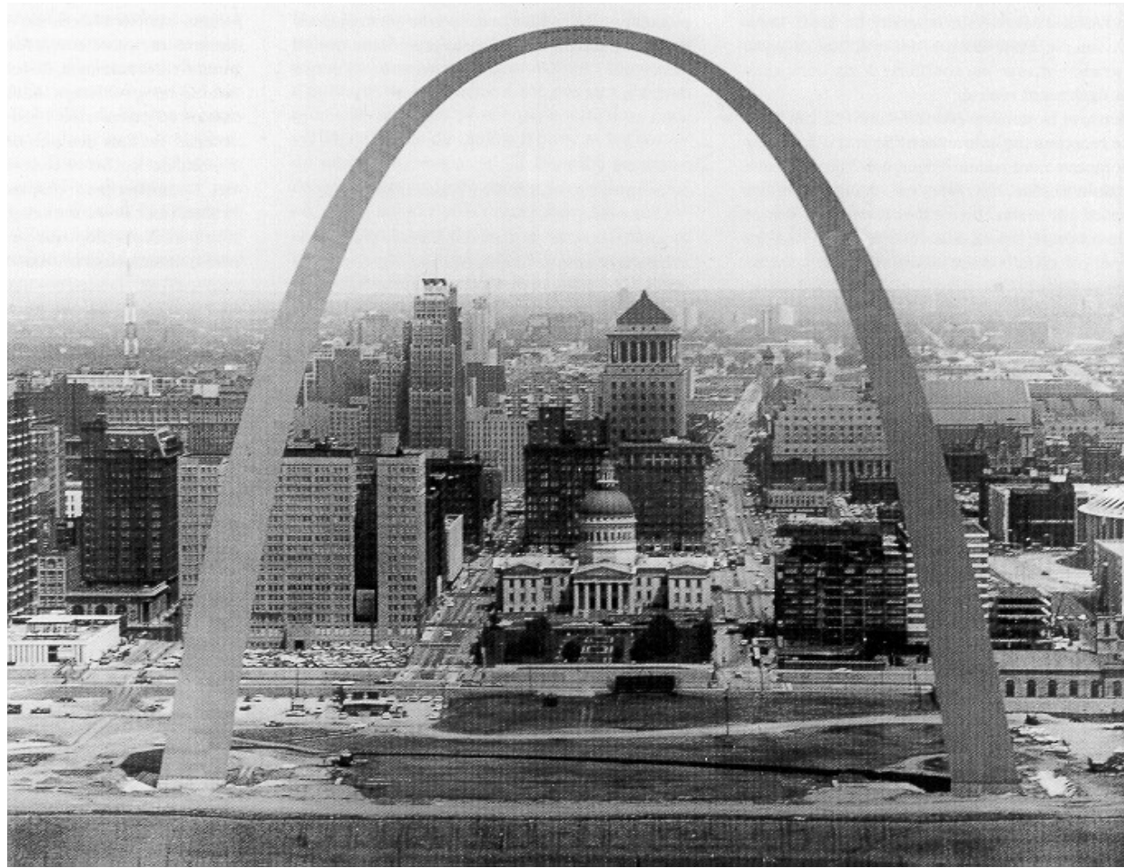
Arc de St. Louis, 1965, arch. E. Saarinen, ing. F. N. Severud ( l=192\text{m} f=192\text{m} , l/f=1.00 )
